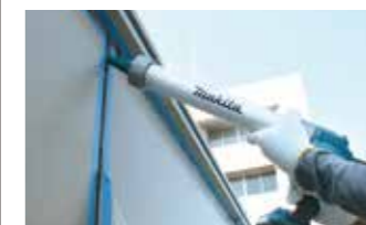
For Sealing work with two-component system
