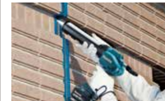
For Bonding of external wall, window frame.
