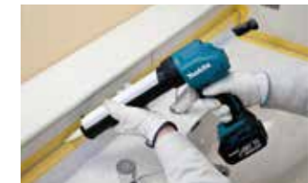
For Water section and Interior finishing
